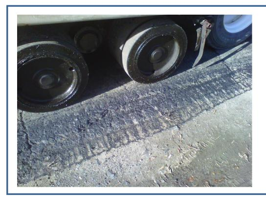
HMA paving operations using conventional tack coats are subject to tire tracking issues. Truck tires, paver tracks and other vehicles that cross any tacked surface can wreak havoc on adjacent areas like driveways and concrete bridge decks. NTCRS-1hM has been formulated to eliminate tire tracking while providing fast breaking speed and the good bond required between HMA layers.
