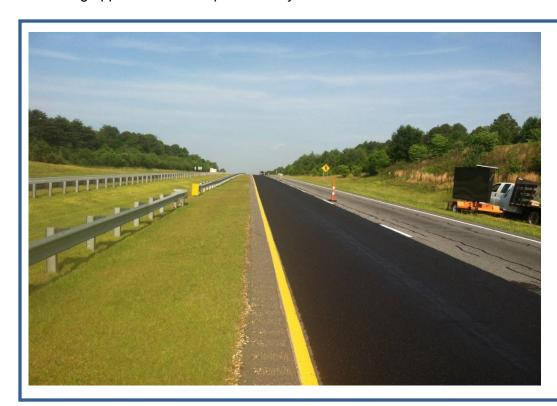
CQS-1hLM emulsion is blended with the chosen aggregate and placed as a pavement preservation treatment to seal pavement surfaces, renew surface texture to improve skid resistance, and is a cost effective way to extend the service life of an existing pavement. Micro surfacing can also be used to correct minor wheel path rutting prior to full lane width applications.
